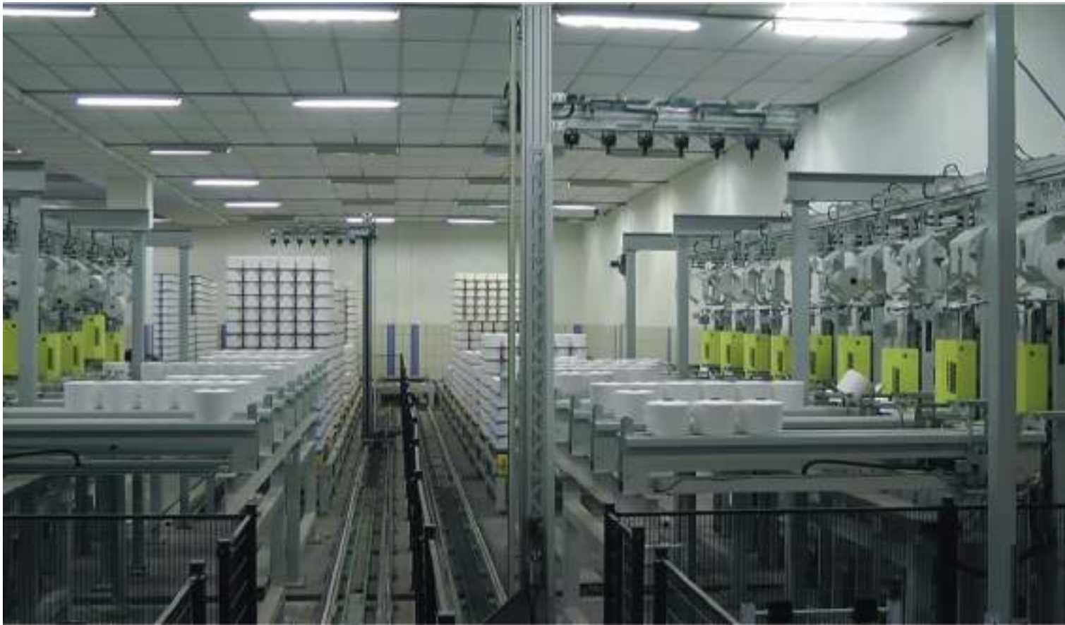
Central palletiser at Neuenhauser
